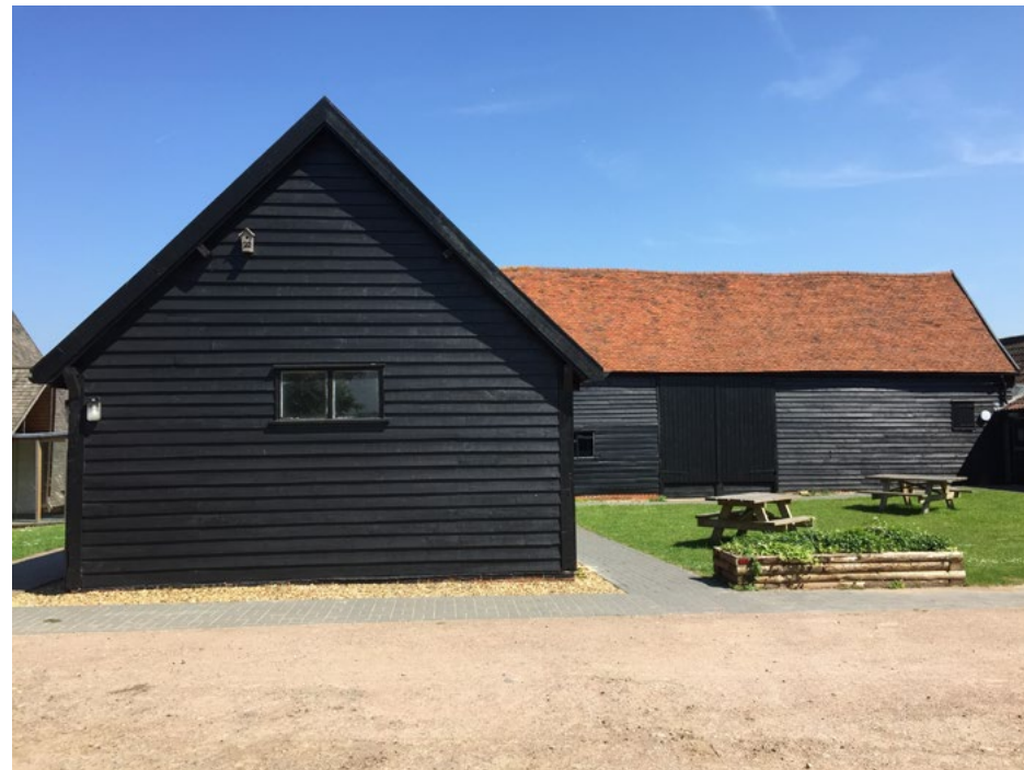
Grade II listed barn at Thames Chase Community Forest
