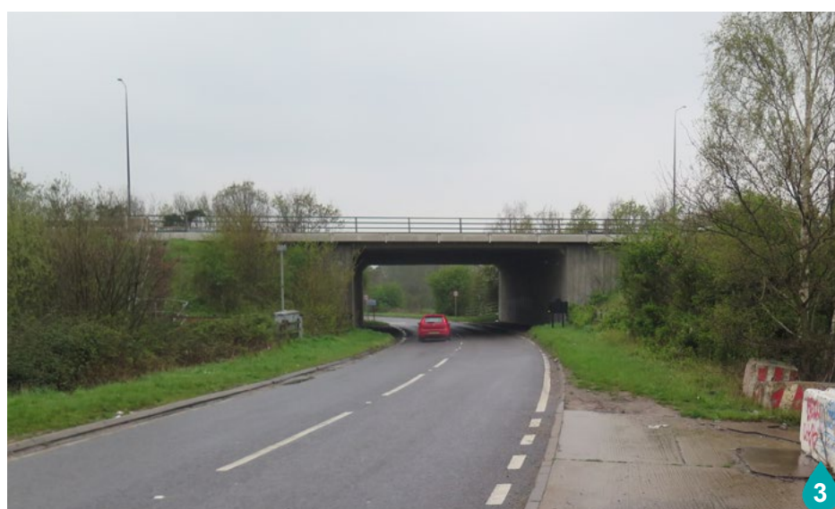
Dennis Road showing M25 overbridge
