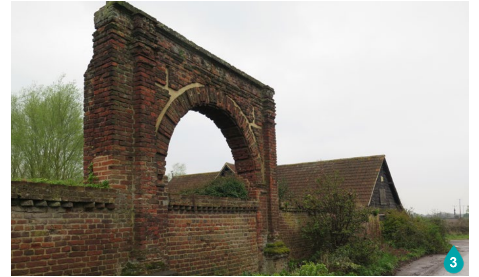
Grade II Listed former gateway at Groves Barns
