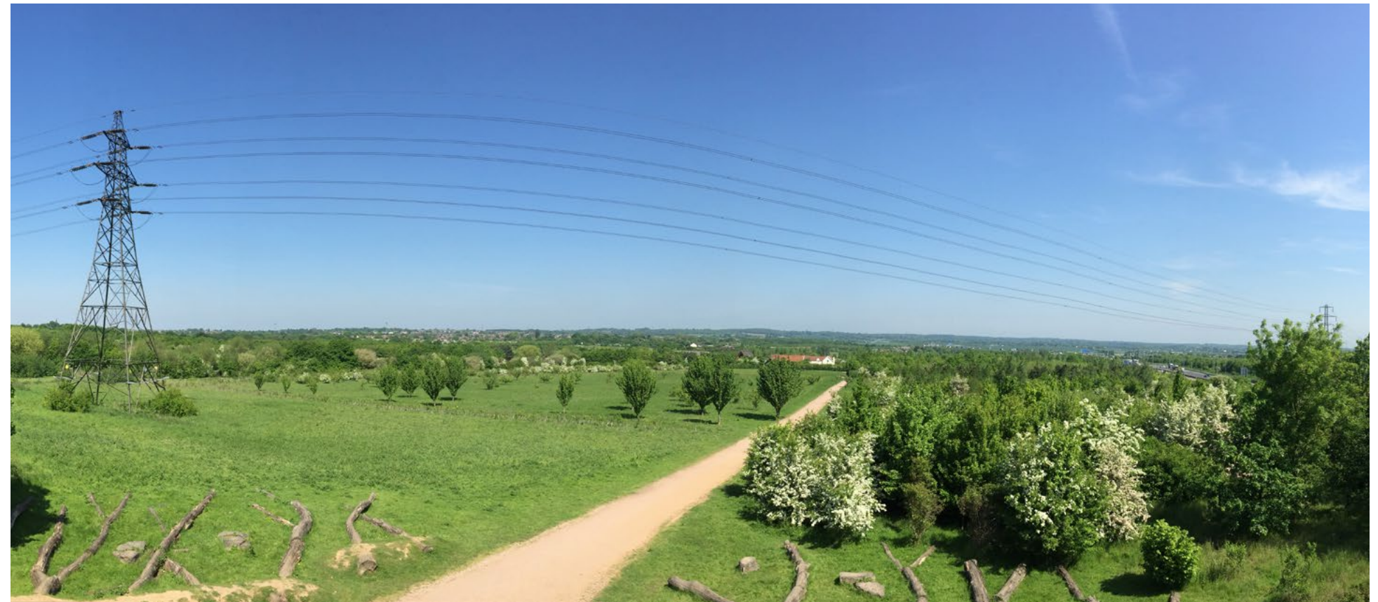
Existing pylons within Thames Chase Forest
