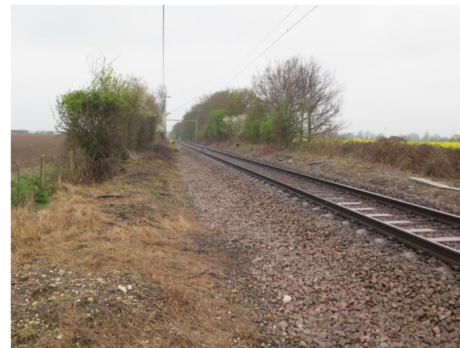
Existing WCH route crosses London Tilbury and Southend Railway railway tracks
