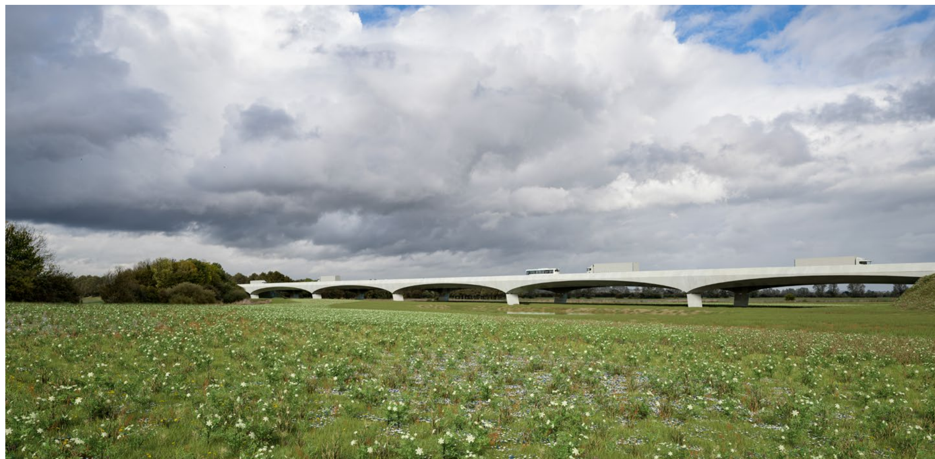
Illustrative view looking at the Mardyke and Orsett Fen Viaducts from the Mardyke trail (BR219)
